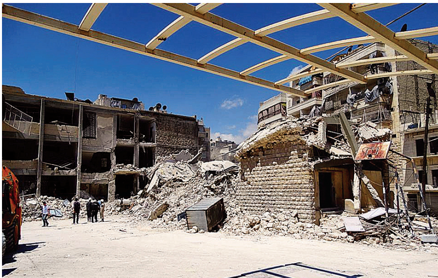
PHOTO: The attacks on the Ain Jalout School in Aleppo destroyed more than 60 percent of the building. (A Press Statement on the Targeting of Two Schools in Damascus and Aleppo “Imprint of Hope Soaked with Blood,” VDC/Photo by Abdullah Badawi, 2014)
